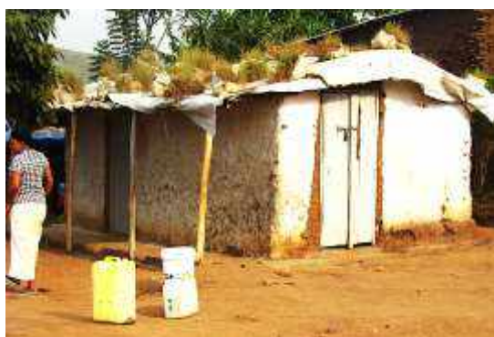
Figure 3. 'Roof Top Gardens', a '3 in 1 climate change adaptation measure' to hold roofs against strong winds,
