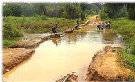
Figure 11: Broken bridge due to flooding
